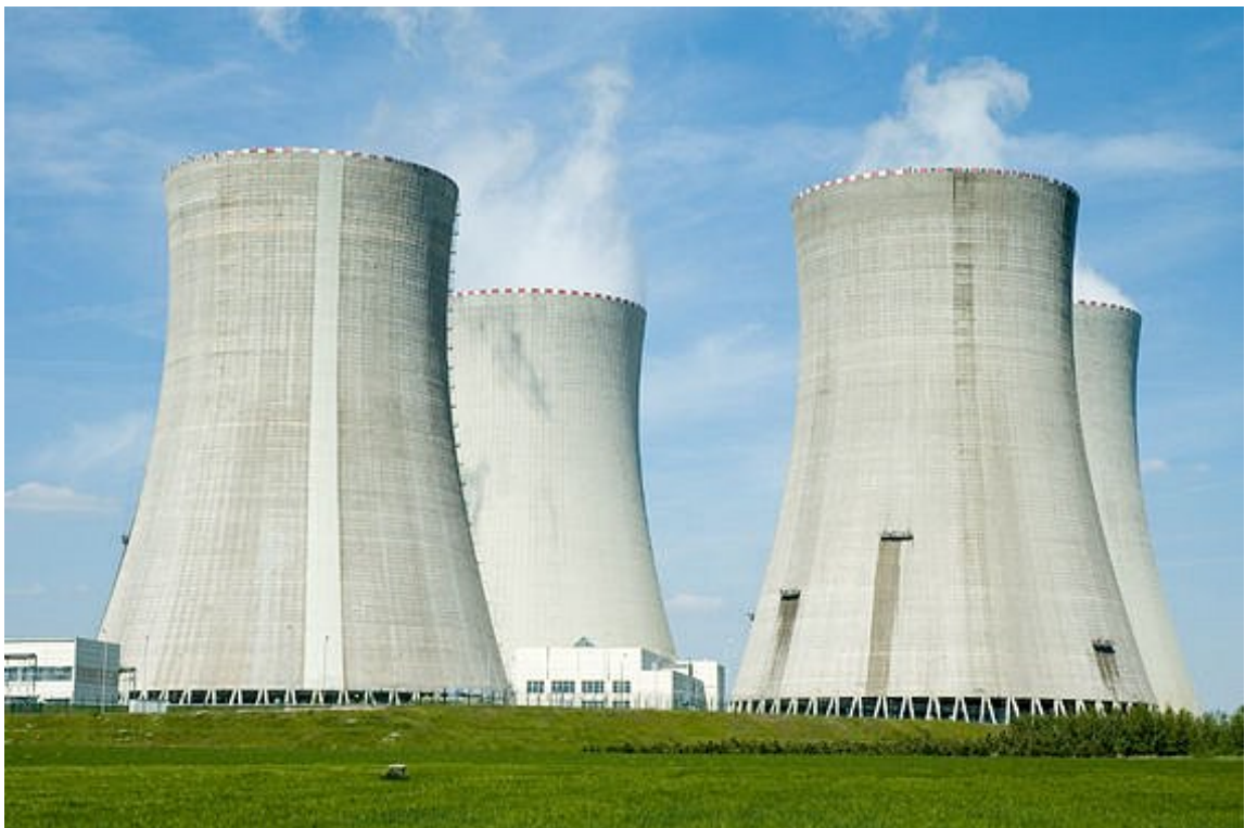
Figure 1: Typical cooling tower
